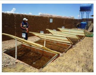
**Fig. 6:** Composting trenches for treatment of the faecal matter (source: Andersson 2011)
